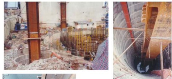
Steel stanchion (column) placed on top of the bore pile as support for top-down basement as well as permanent column for future structure
