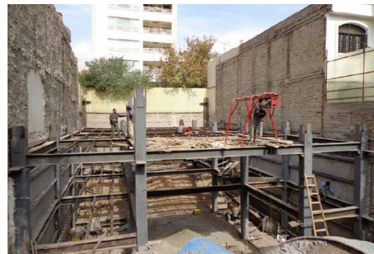
Excavation and construction of the basement slab using double-bit arrangement
